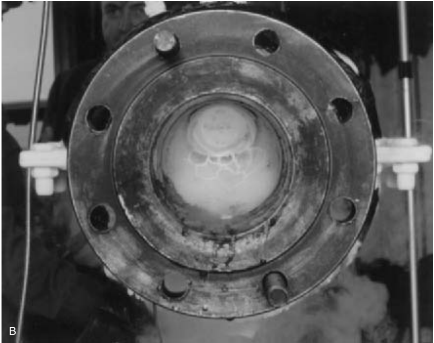
FIGURE B14.9b End view in which actual freeze plug can be seen. ( Team, Inc., Alvin, TX )
